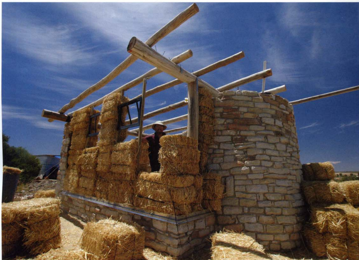
Gatehouse of the Nieuvoudteville Caravan site upgrade project.
