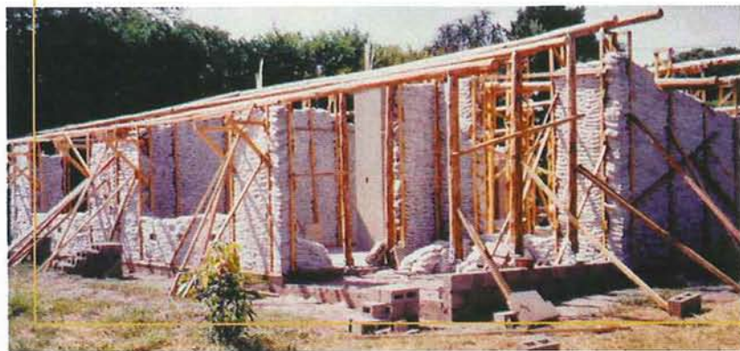
Above: A modern Eco design house uses bags filled with sand forming strong, sturdy walls.
