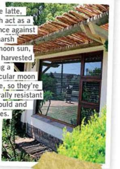
A natural plaster of cow dung, clay water, sand and building lime is mixed on-site.
