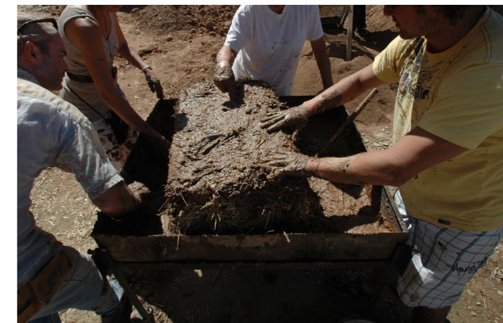
Working together to pre-plaster a straw bale. Barrydale, Western Cape. Photograph courtesy of Ansgar Von Oertzen
