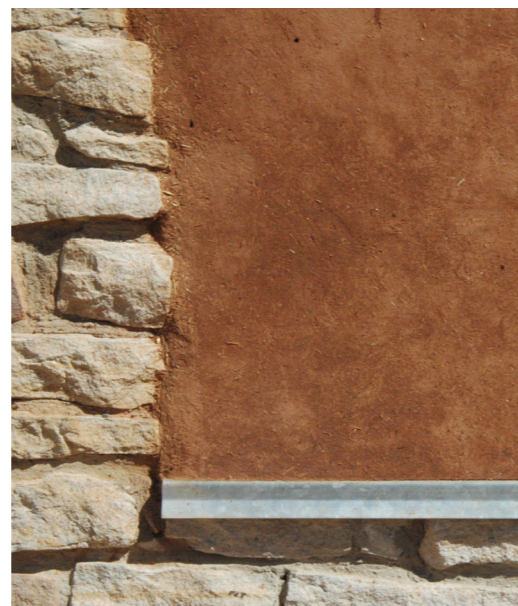
Strawbale wall with earthen plaster, Nieuwoudtville, Northern Cape
