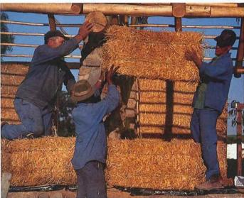
Skillful Means, a Californian-based architectural and construction firm active in strawbale construction, states: "A plastered bale wall provides a good barrier against air and water... because bale walls are highly fire resistant, this structural system comes with its own fire proofing." Straw-bales are a waste product and using them will not damage the environment or waste resources.
